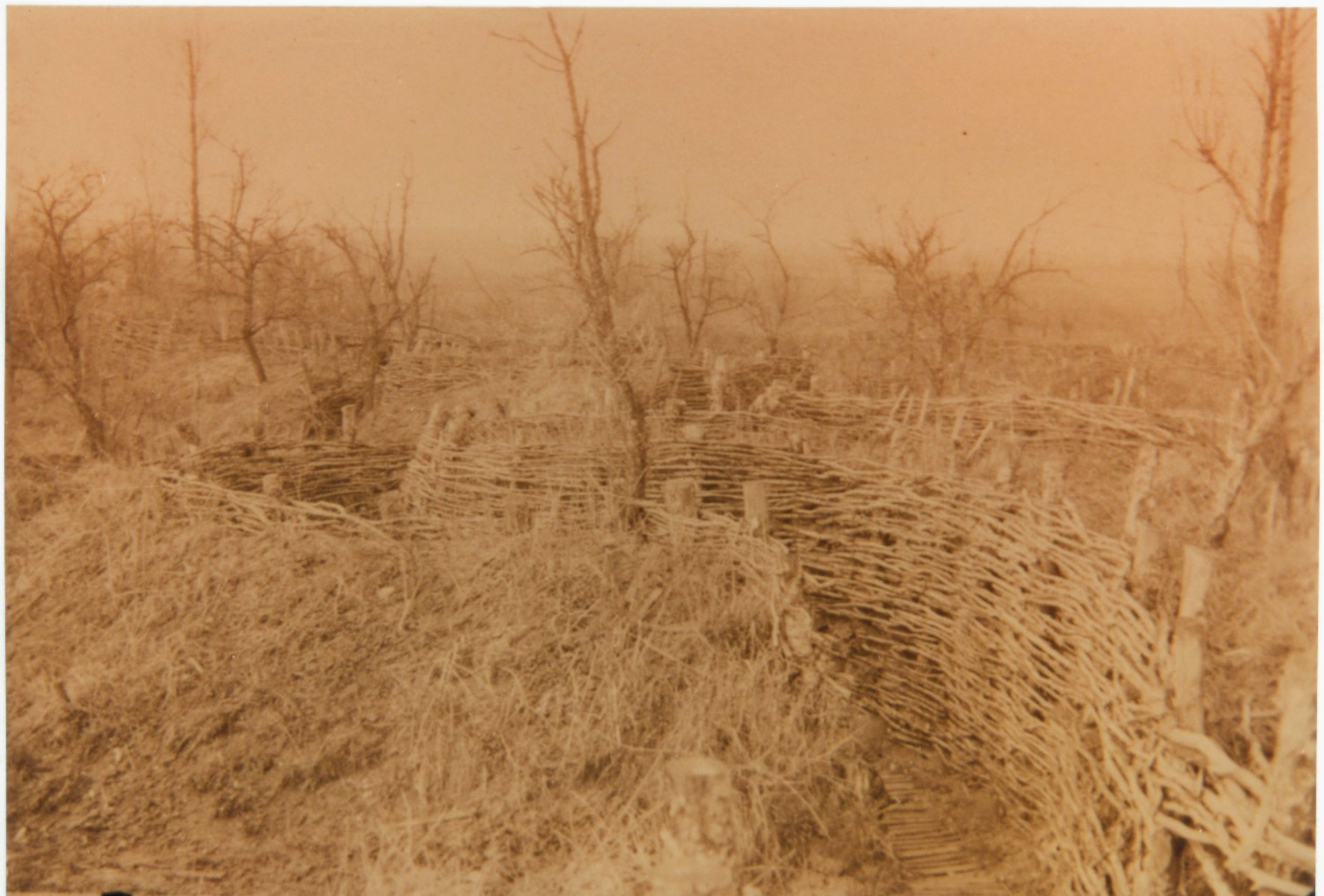
German Trenches, near Marcheville. Note method of construction in swampy ground.
