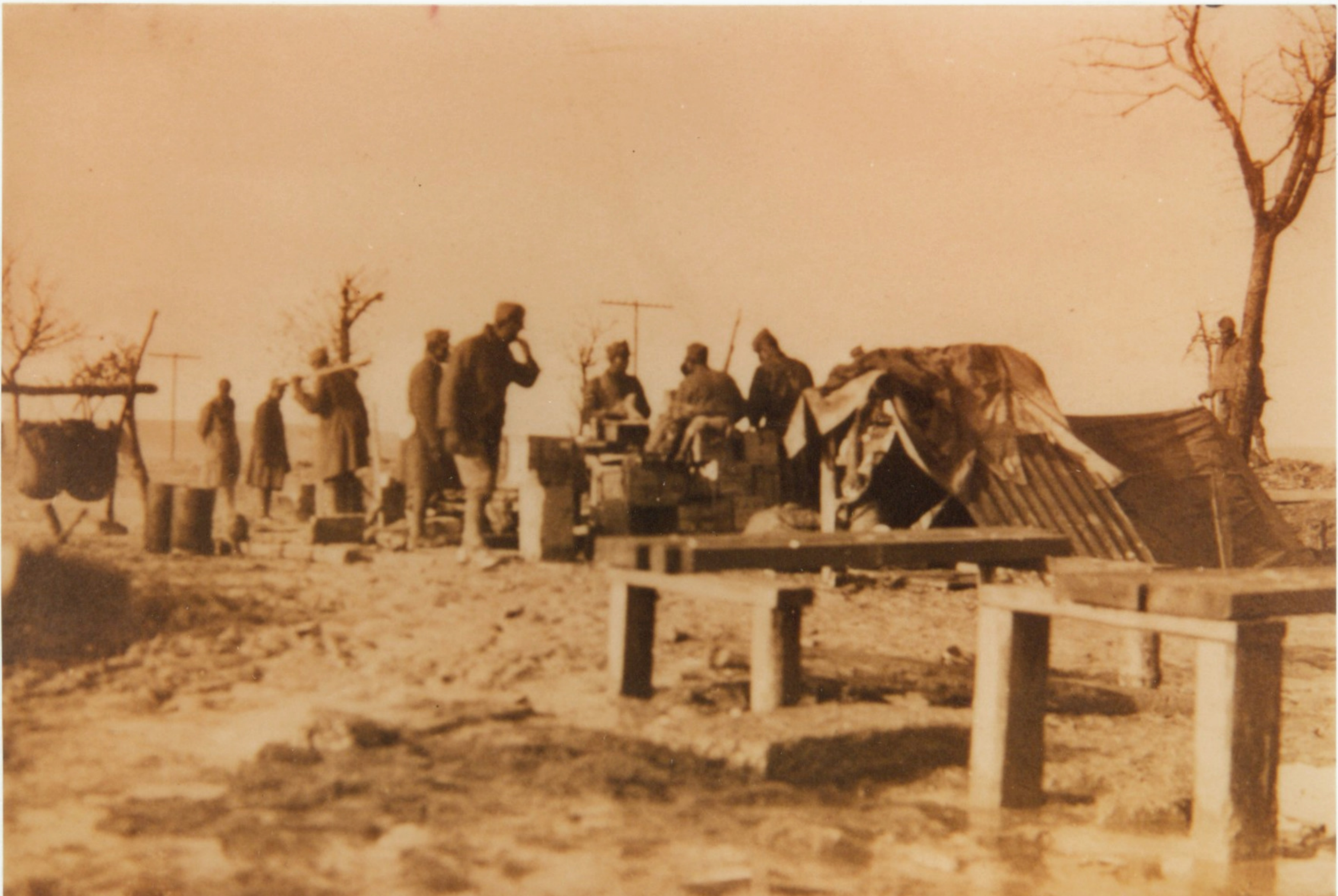
Colored Engineer labor troops engaged on road work in the vicinity of Arava Court Verdun-Pont-a-Musee
