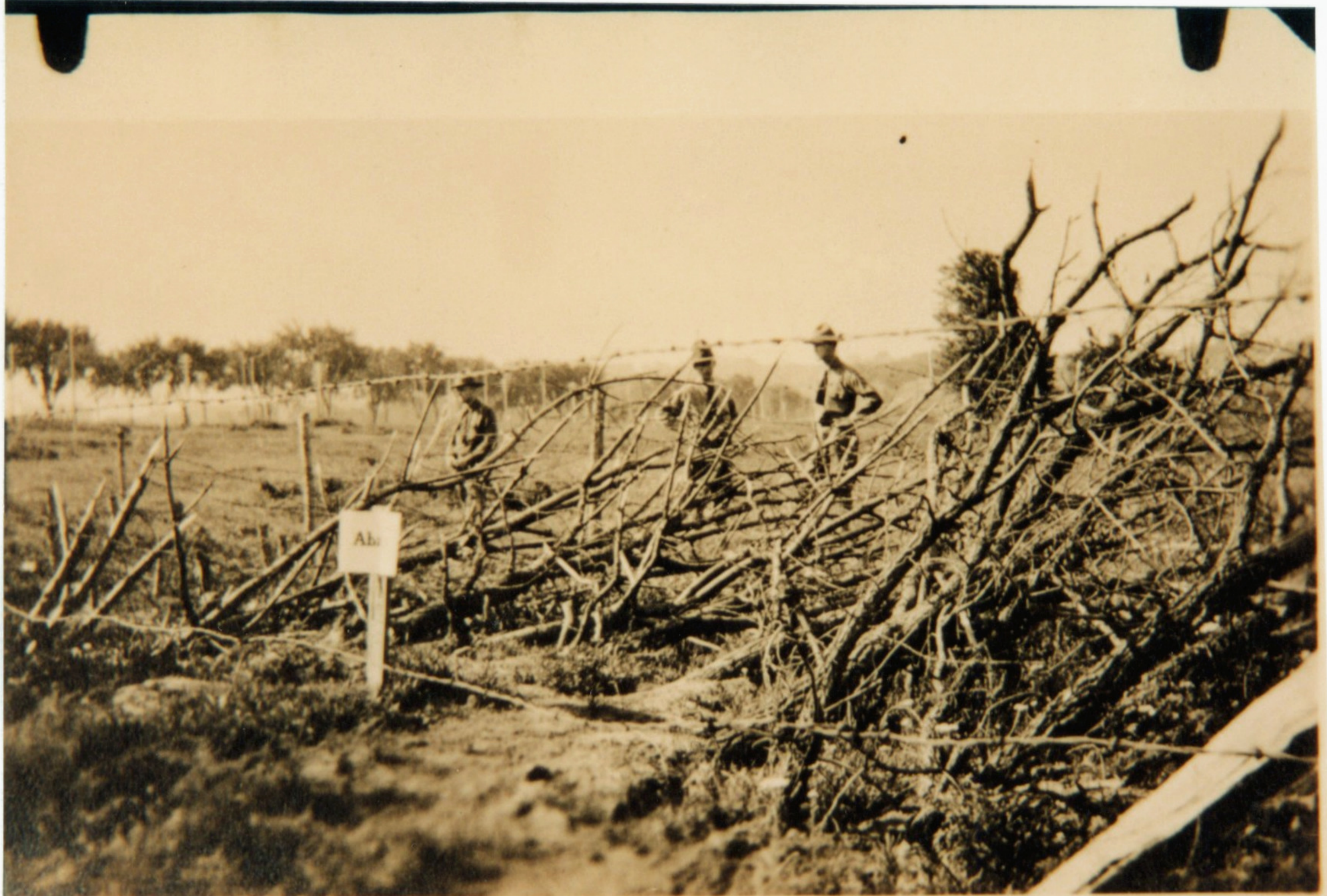
Types of construction for Abatis, Fort Leavenworth, Kansas, E.R.O.T.C. Summer - 1917
