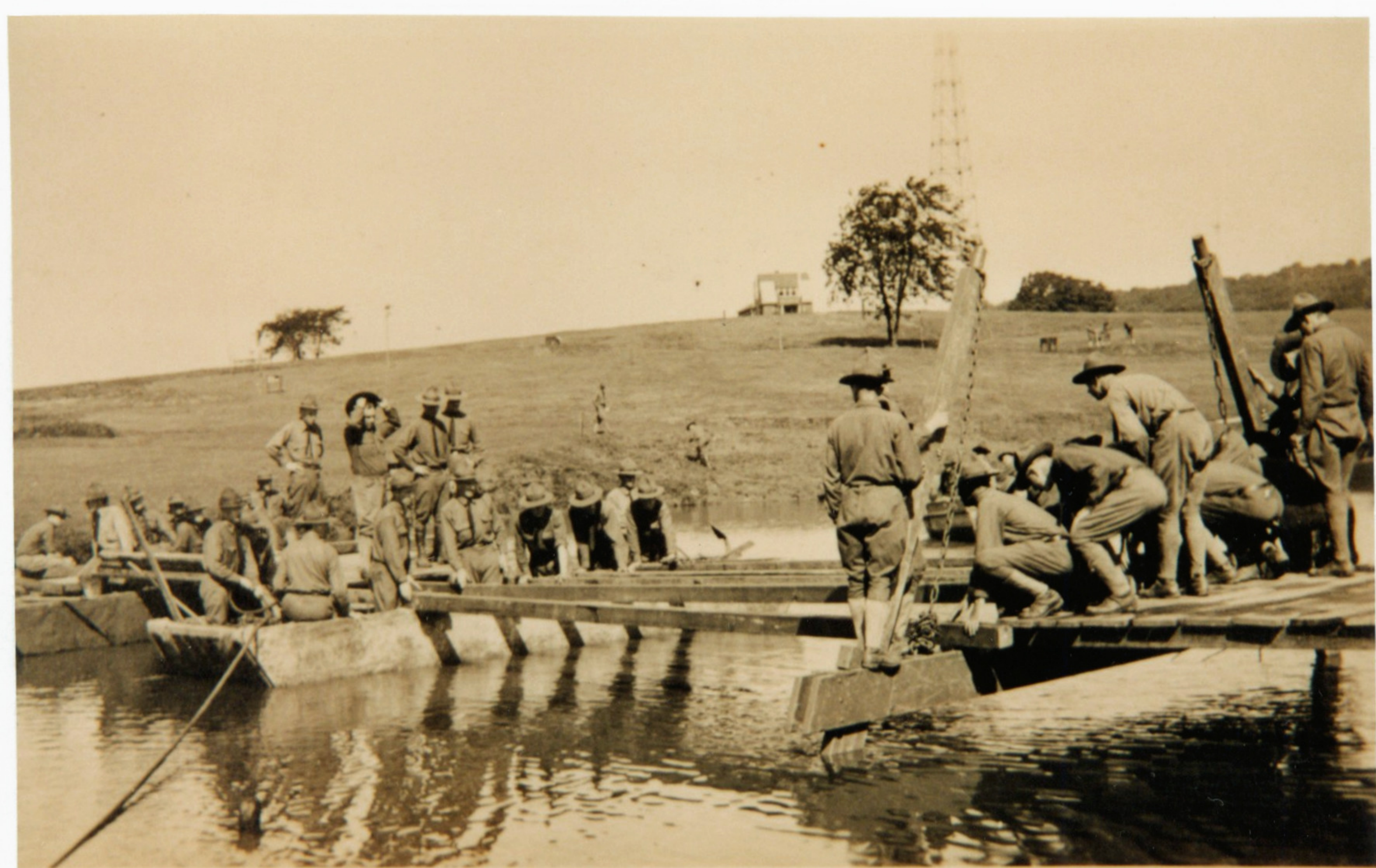
E. R. O. T. C. constructing pontoon bridge of "Knock-
