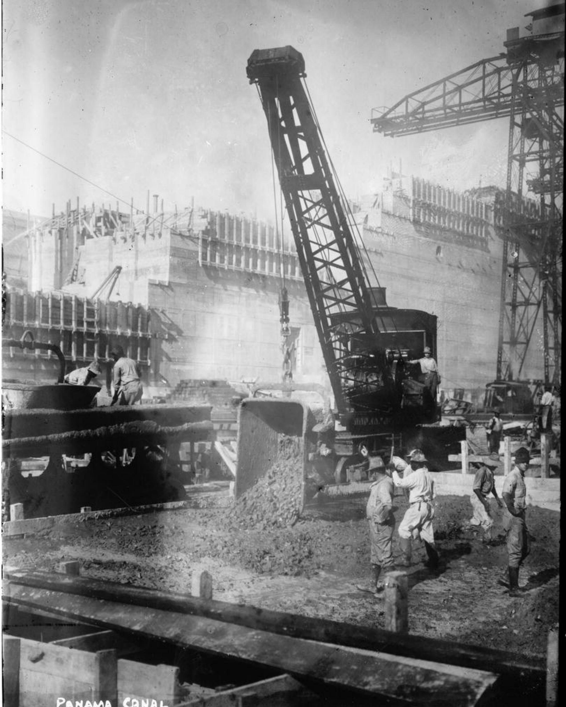
33-L.6 - Pedro Miguel Locks. Auxiliary Crane Dumping Concrete
